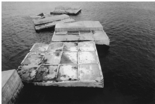
FIG. 2. Sliding of Caisson (Courtesy of S. Takahashi)
